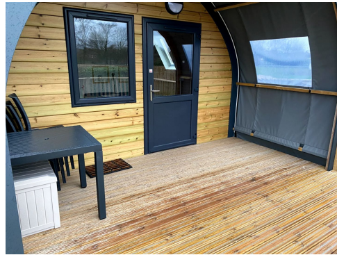
The front door has a level threshold.
